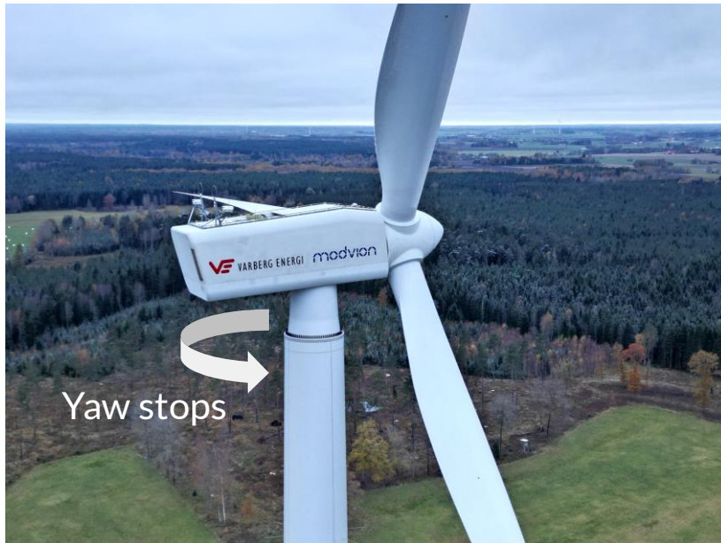
Real wind turbine
